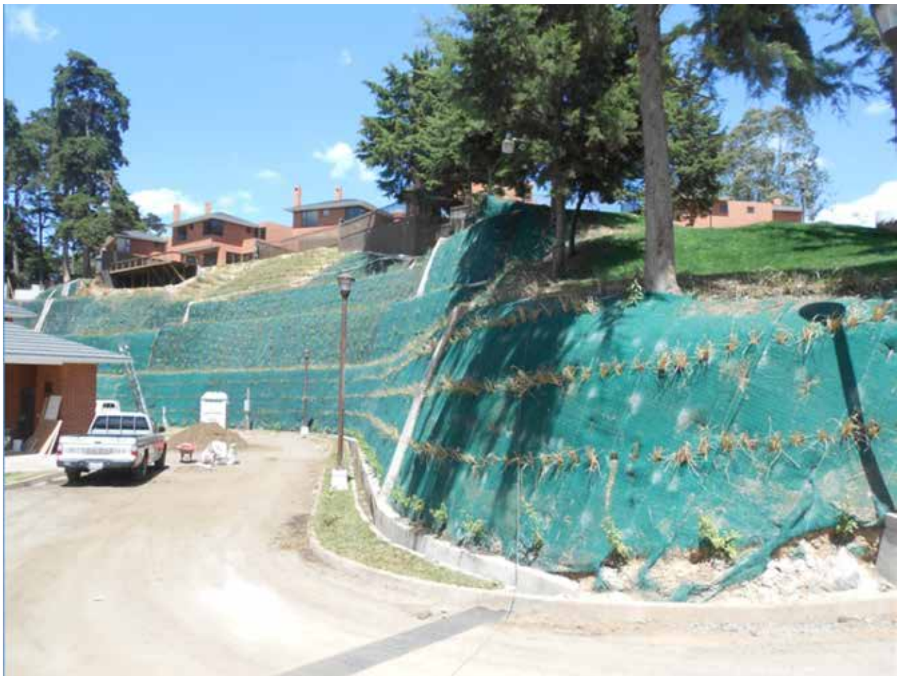
Very steep Batters with geofabrics
