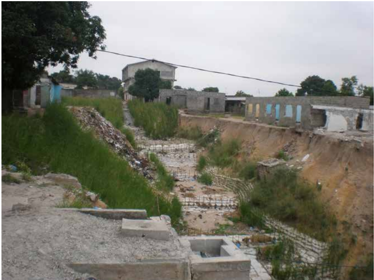
Excellent vetiver growth and the ravine stabilized
