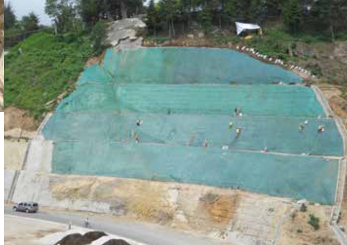
Very steep Batters with geofabrics
