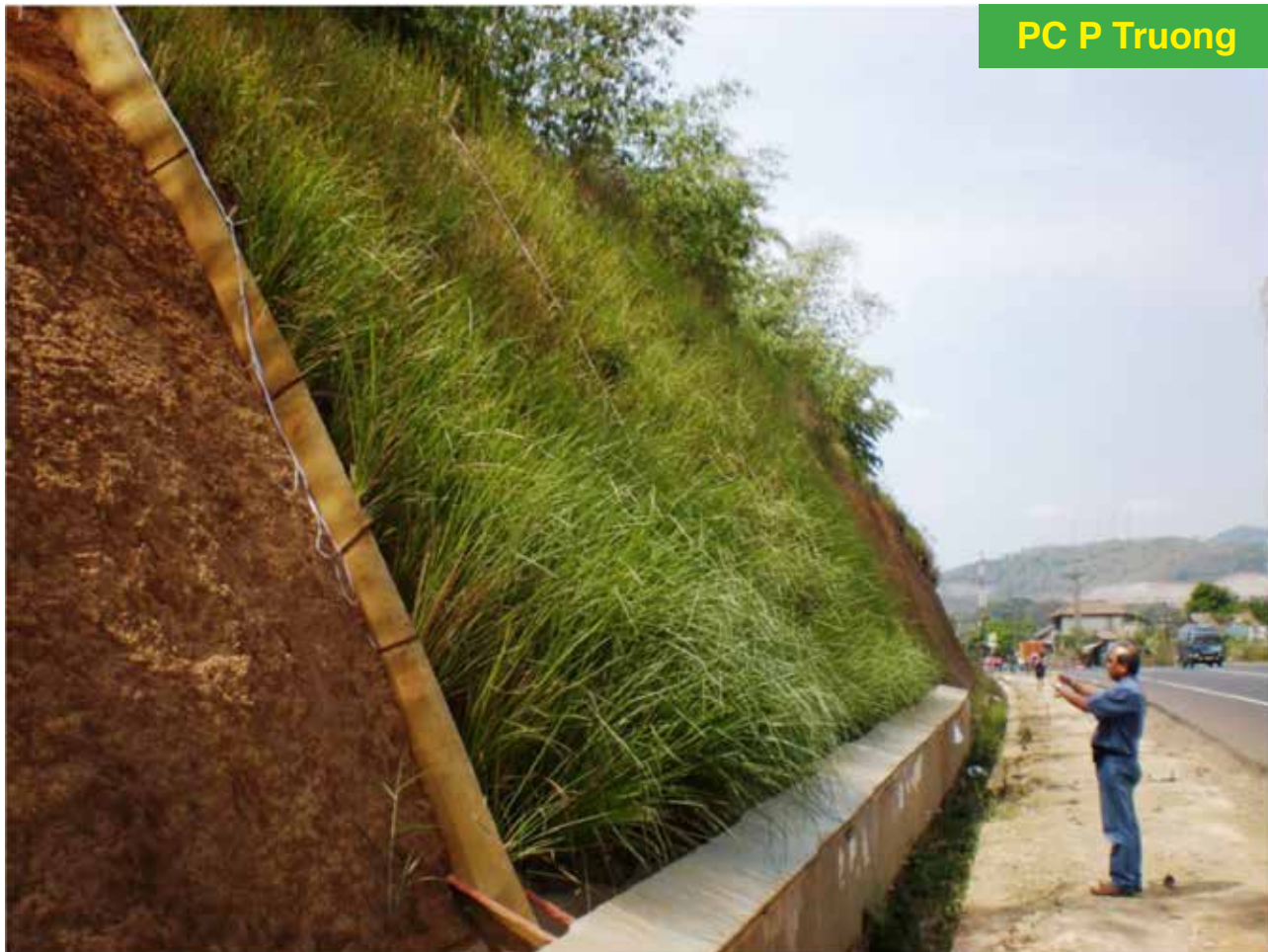
Very steep, 72° slope on highly erodible red volcanic soil
