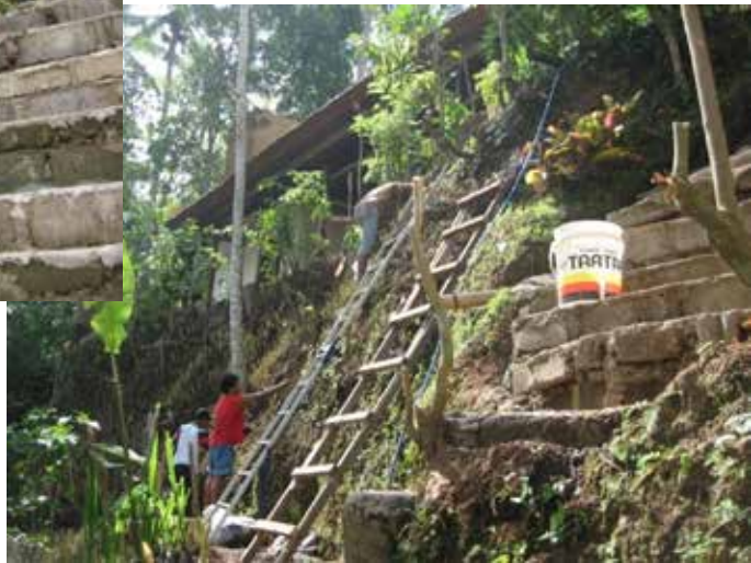
Planting vetiver using long ladders
